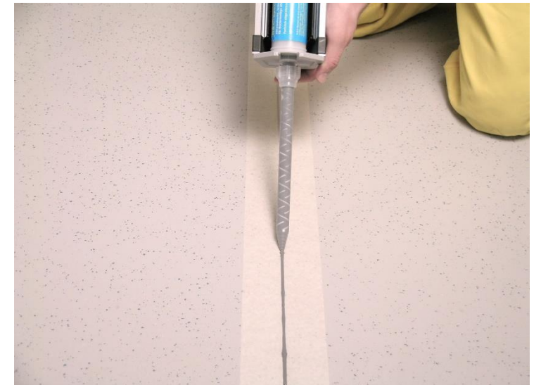
3 - Apply NEW ELASTJOINT 2 inside the joint
