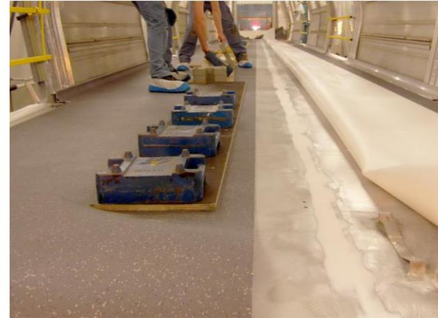
b) Cut the floor in the required dimensions.
